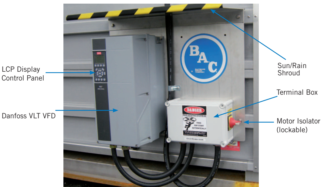
Figure 2. BAC Intelvap Controller Assembly
